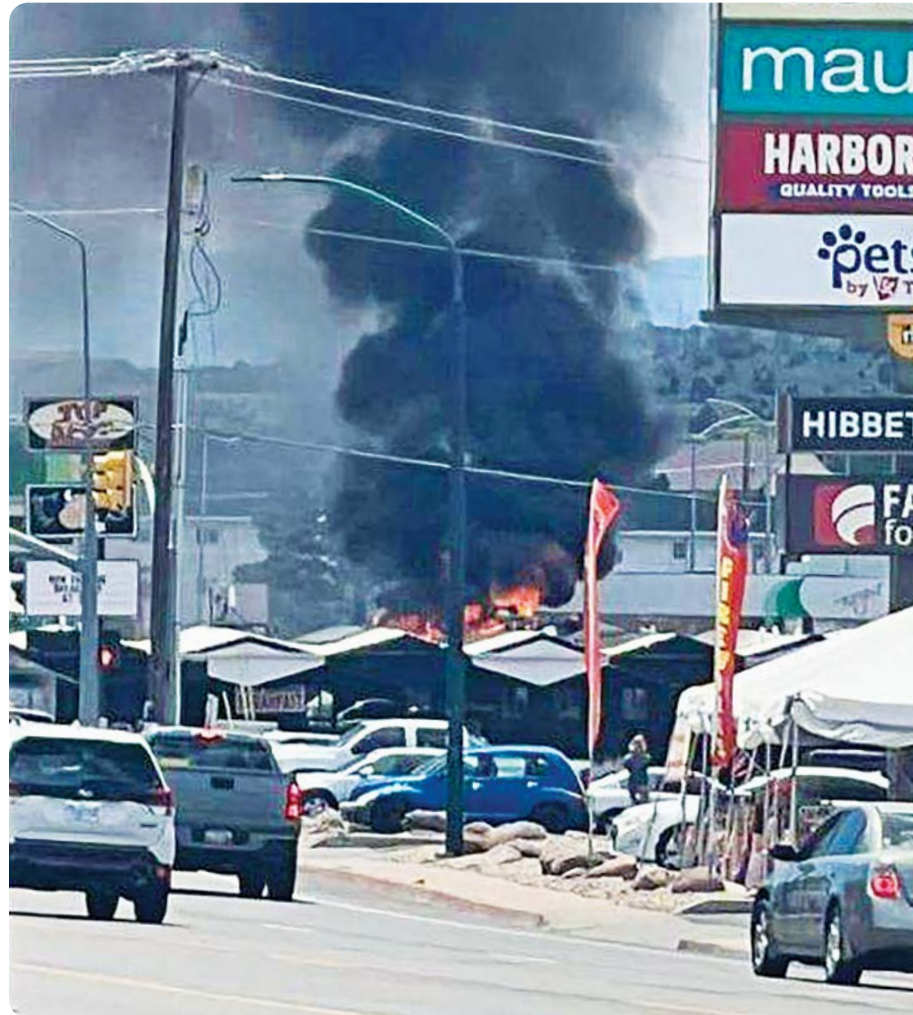
Flames erupt from the roof of Top Spot in Cedar City. A fire crew arrived in time to save the structure from further and permanent damage.
