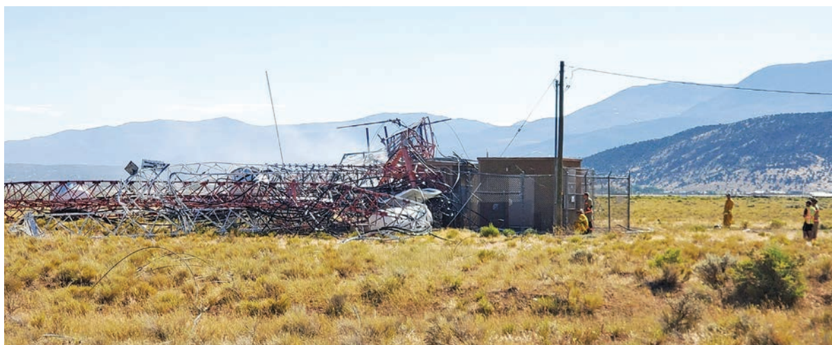
THE COMMUNICATION TOWER which the airplane struck was completely destroyed.
