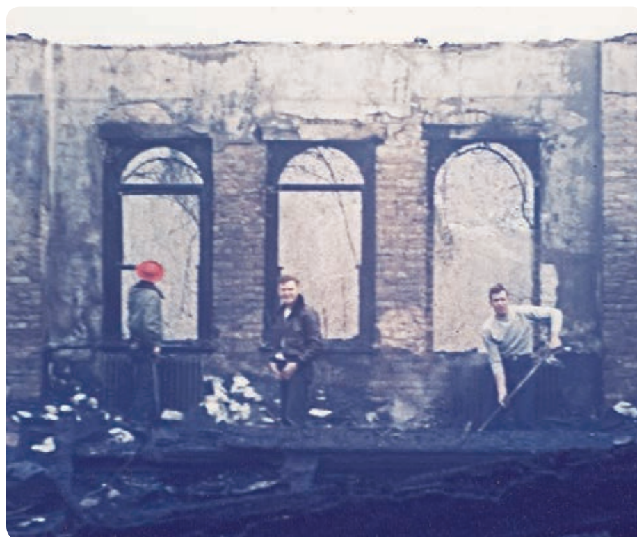
After the clean-up, the main structure was saved enough to be able to remodel it the following year and it became the new Administration Building.
