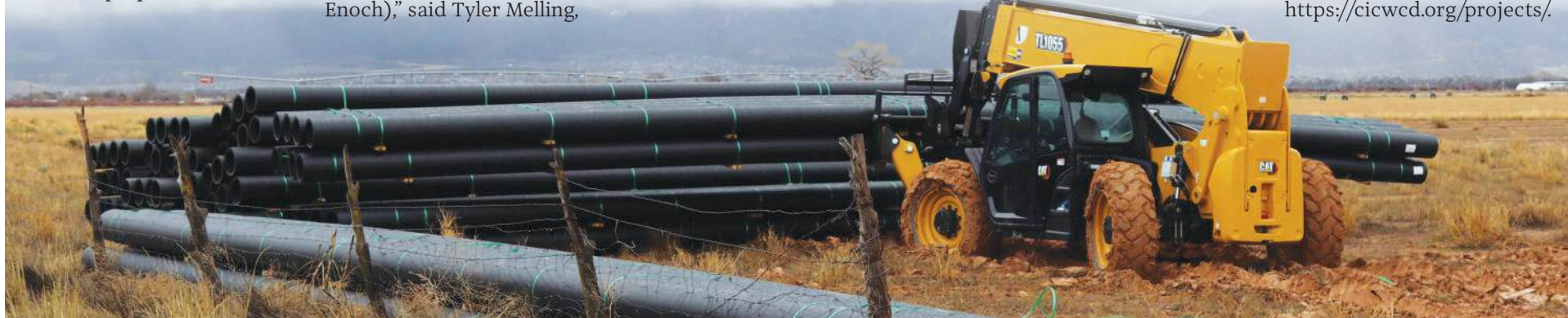
Water Pipe: Pipe delivery for the 4000 N waterline which will help increase efficiency of the District’s water system.
