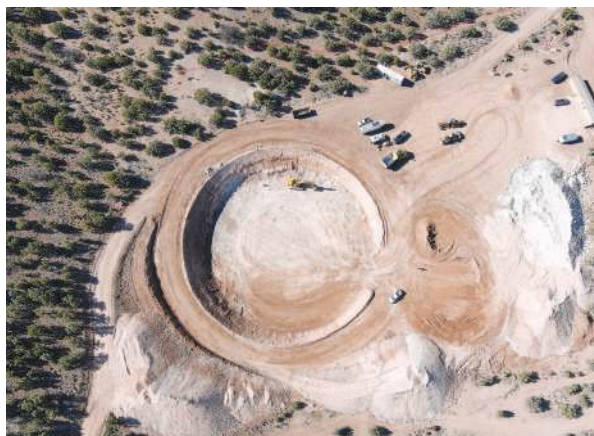
Aerial View of Tank Site: The 4-million-gallon water tank at Eight-mile Hills is under construction and will provide greater water storage capacity for the Cedar Valley
